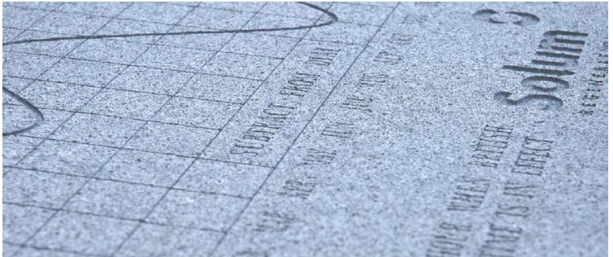
**Figure 7 Example of sandblasted text onto concrete**
